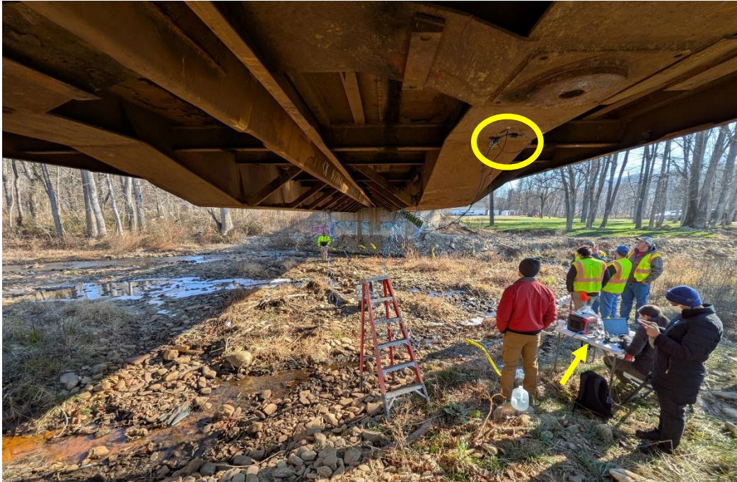
Figure 10. Measurement location at the west end (yellow circle) and arrangement of the data acquisition system (yellow arrow)
