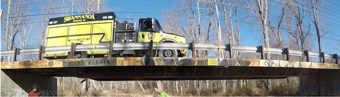
Figure 20. Truck positioned at the 30 ft marker creates maximum strain at the tapered section
