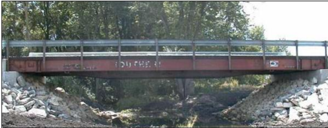
Figure 4. Permanent RRFC Bridge in Iowa Made from a 56' Long V-Deck Flatcar (from TR-498) Note the short span and different cross section relative to the WNC temporary RRFC bridges.
