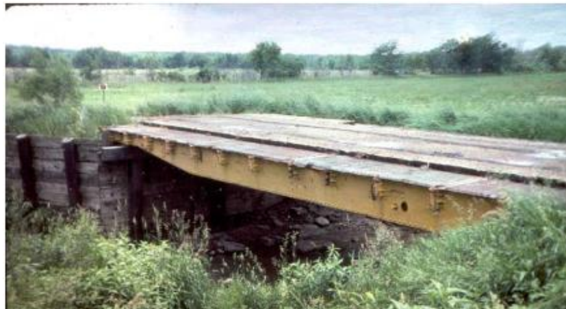
Figure 3. Permanent RRFC Bridge with a Short Span, Timber Deck, and no Railings on an Unimproved Road in Iowa (reproduced from TR-421)
