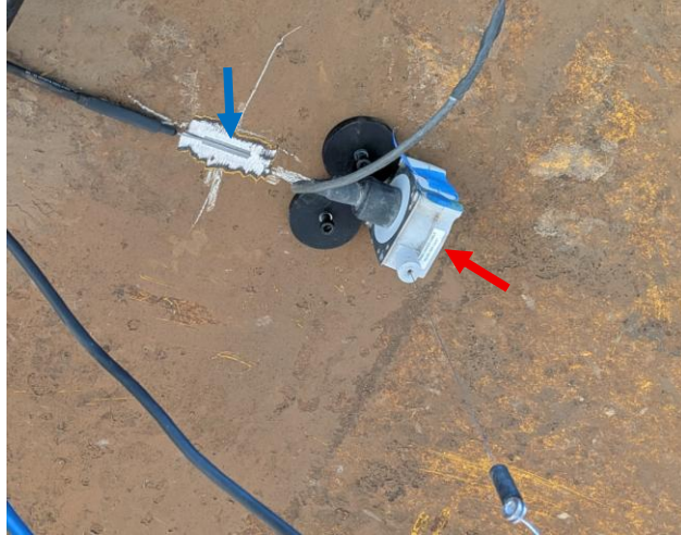
Figure 8. Strain gage (blue arrow) and string potentiometer (red arrow) at a typical measurement location
