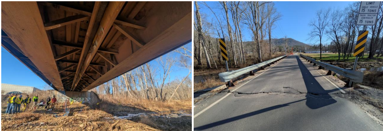
Figure 7. Temporary railcar bridge in Swannanoa, NC (Buncombe #203)
