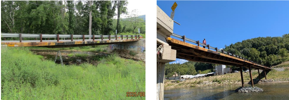
Figure 1. Temporary RRFC bridges in WNC in Swannanoa (left) and near Burnsville (right)
